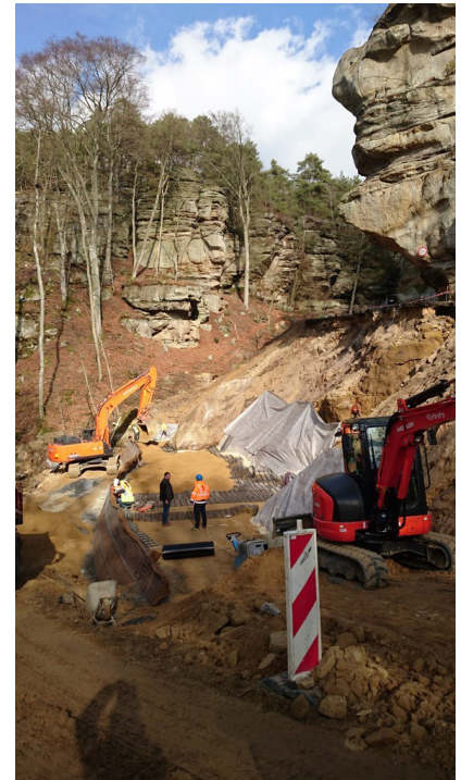
Figure 11: Stabilisation system under construction.
